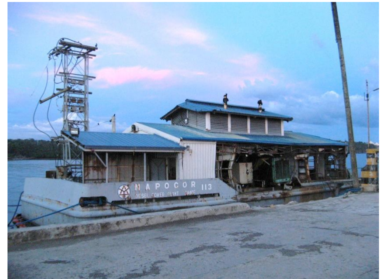
Fig: Destroyed diesel power barge, Lazi, Siquijor. May 2013.
