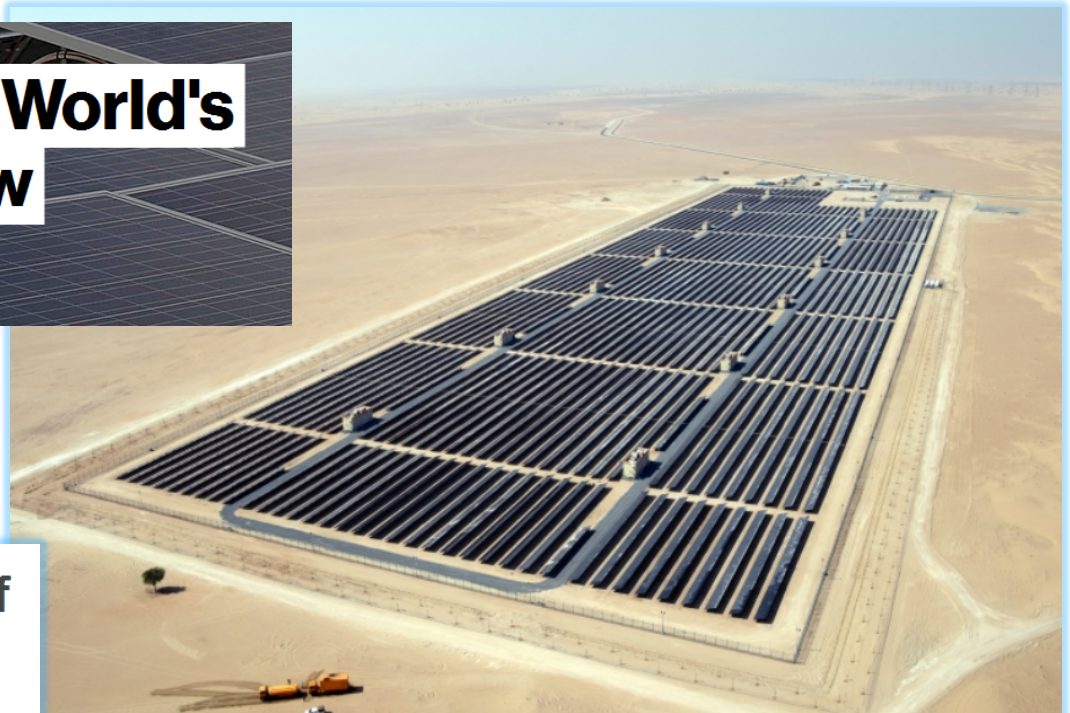
Phase 1 of the Mohammed bin Rashid Al Maktoum Solar Park. Source: First Solar.
