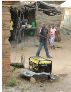
Small diesel generator to power little energy kiosks – Extreme Nord, Cameroon (Cader, 2014).
