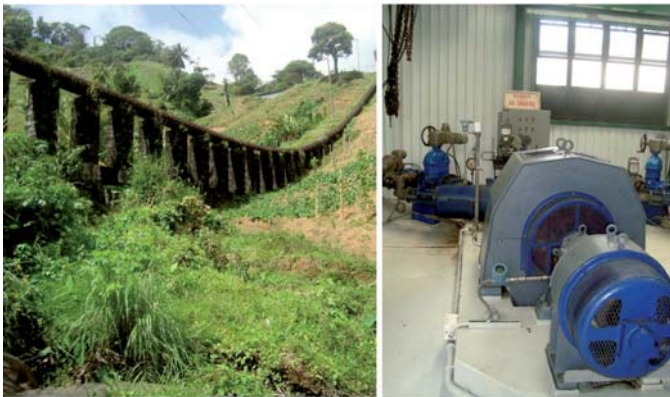
Figure 2.8: Picture of small hydro plant on St. Vincent, St. Vincent and the Grenadines, own photo source
