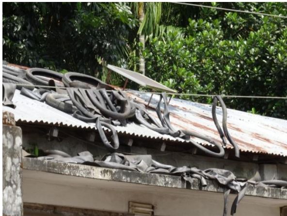
Solar home system & distribution grid, Hatiya Island Bangladesh (Bertheau, 2014).
