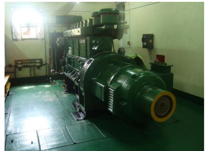
Abb. 4: Diesel GenSet, Lister E 56, Petite Martinique (Blechinger, 2011)
